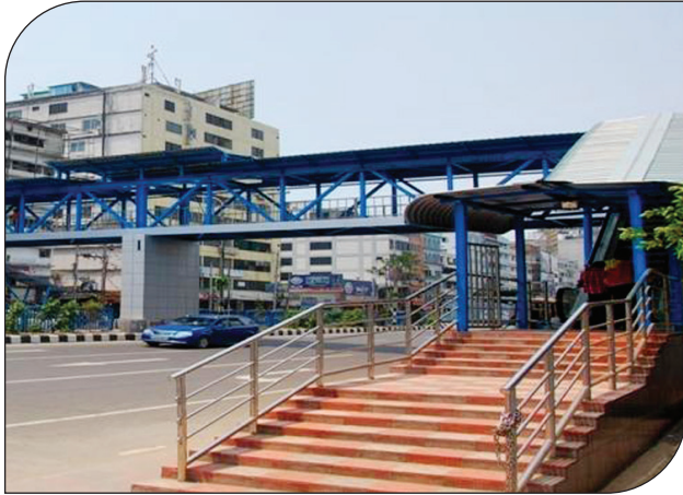
Foot over Bridge/Steel Bridge
