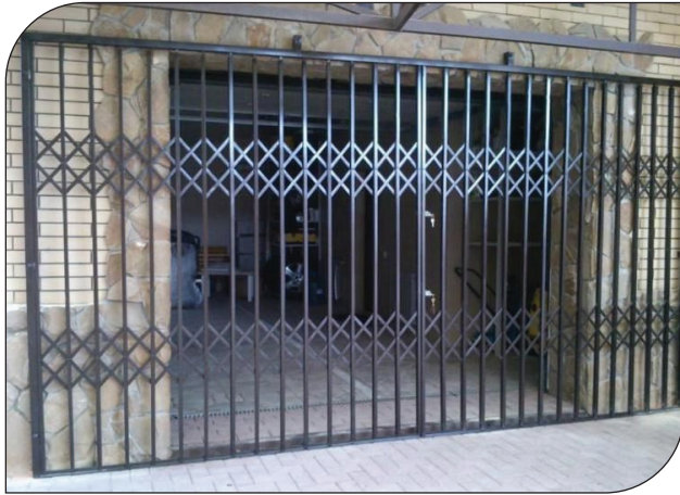
Collapsible Channel Gate
